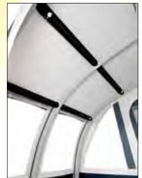
Inside view of the roof tubes
